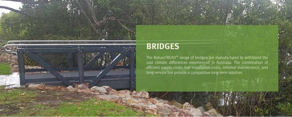
Bridges constructed from traditional materials of timber and steel are increasingly being replaced by FRP bridges. FRP bridges are more cost-effective than their traditional counterparts as they require substantially lower maintenance and replacement. Being lightweight and easily pre-fabricated greatly reduces installation times and eliminates the need for heavy machinery. This further improves cost savings as labour time and equipment operational costs are greatly reduced.
