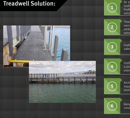
As part of the Treadwell EnviroTREAD<sup>™</sup> range, high performance GratEX<sup>®</sup> FRP Square Mesh grating and ArchitEX<sup>™</sup> FRP Structural Profiles were specified in building the structure as a preferred solution over traditional materials.
